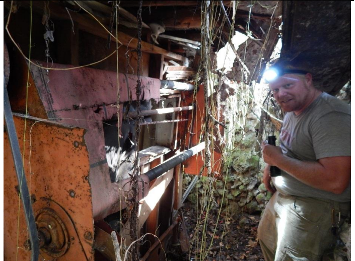
Figure 5 - Ciphering up some repairs on the Cave Elevator
